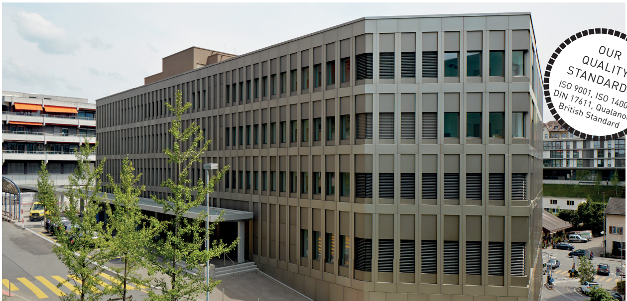
Ophthalmology Clinic of Lucerne Cantonal Hospital in Lucerne, Architecture: Schneider & Schneider Architekten ETH BSA SIA AG, Image: Peter Ruggle
